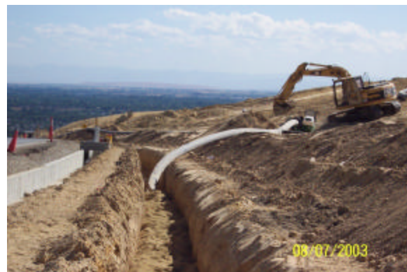
Figure 7 Installation of Header Pipe
