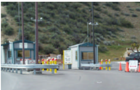
Figure 4 - Welcome to Hidden Hollow Sanitary Landfill
