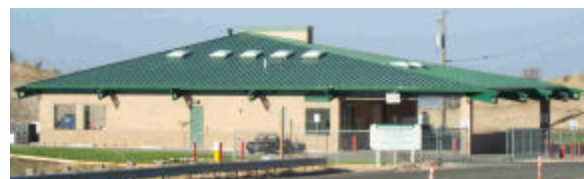
Figure 5 - Ada County's Household Hazardous Materials Collection Facility
