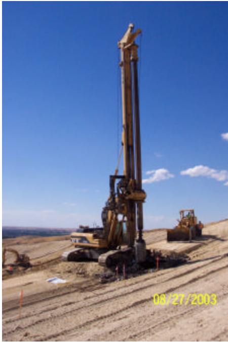
Figure 8 Landfill Gas Drill Rig
