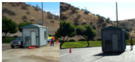
Figure 17 - (left) Access road ready for paving. (right) Paved.
