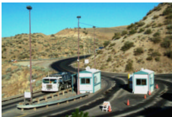
Figure 2 - Hidden Hollow Landfill Gate
