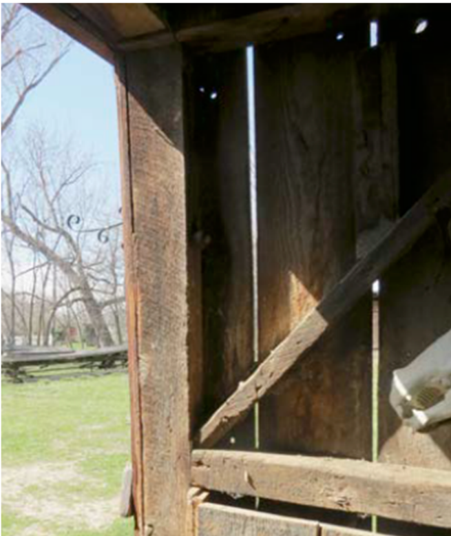
Second Section constructed of milled lumber rather than hewn beams.
