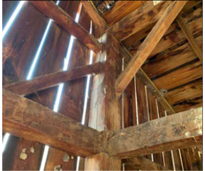
Hand hewn beams with mortise & tenon joinery secured with wooden pegs.
