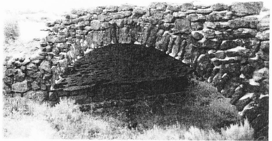
Bridge Field No. 402
