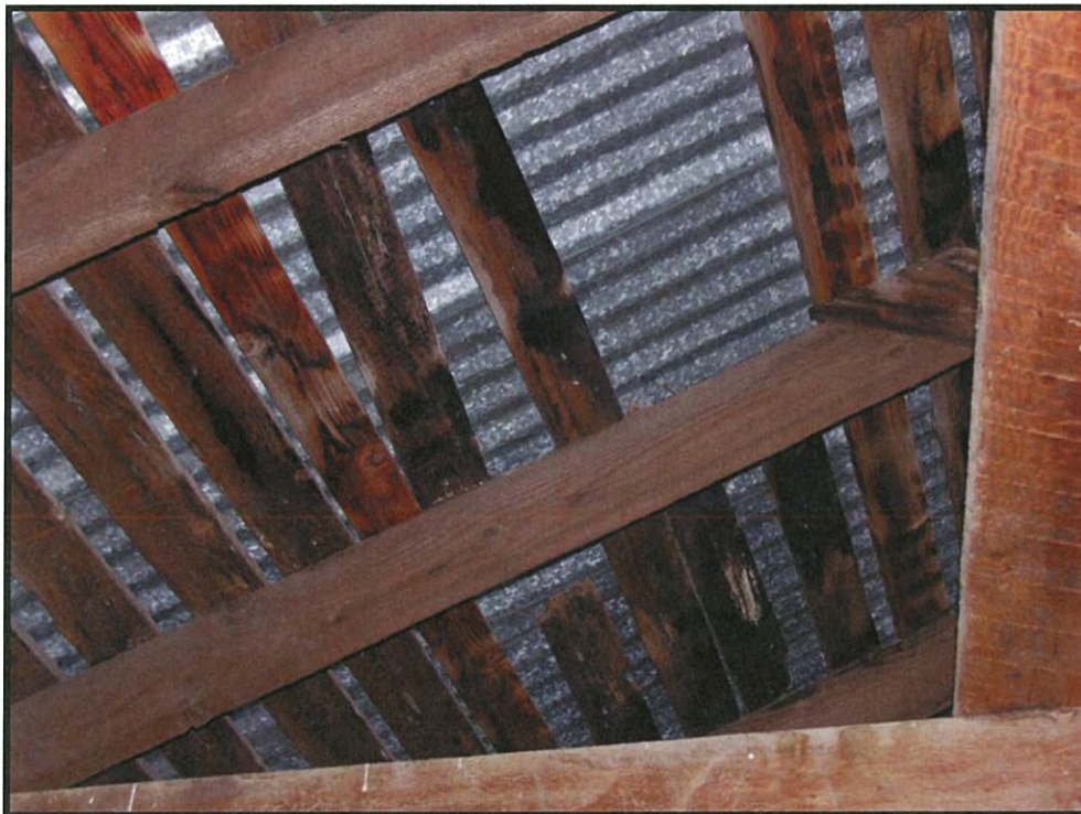
Figure 20. Feature 2, Horse Barn, detail of damage to roof covered by new corrugated metal (DSCN4214; 06/18/2016).
