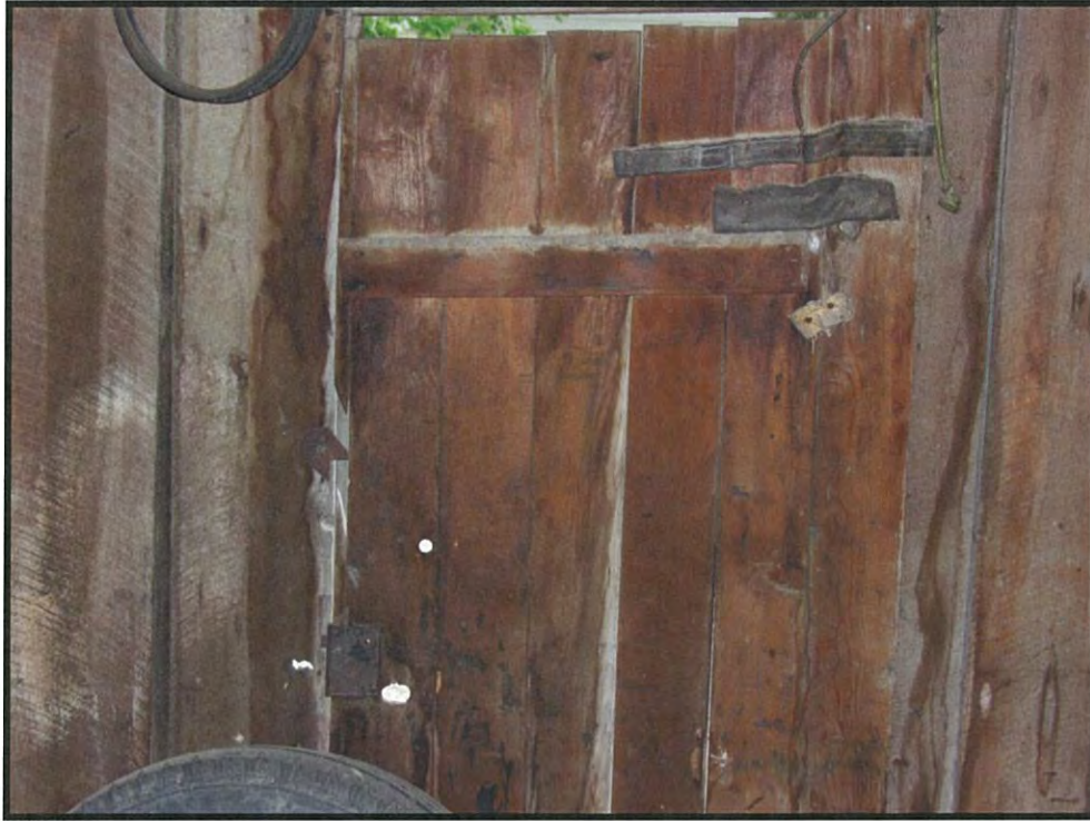
Figure 19. Feature 2, Horse Barn, leather door hinge detail (DSCN4213; 06/18/2016).
