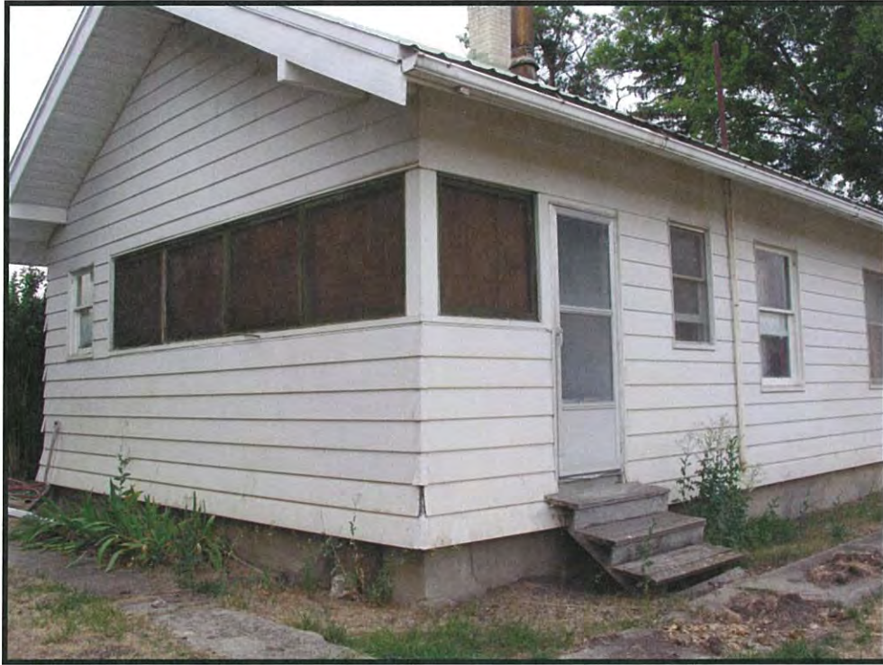
Figure 25. Feature 4, Dwelling, to the southwest showing porch addition (DSCN4236; 06/18/2016).
