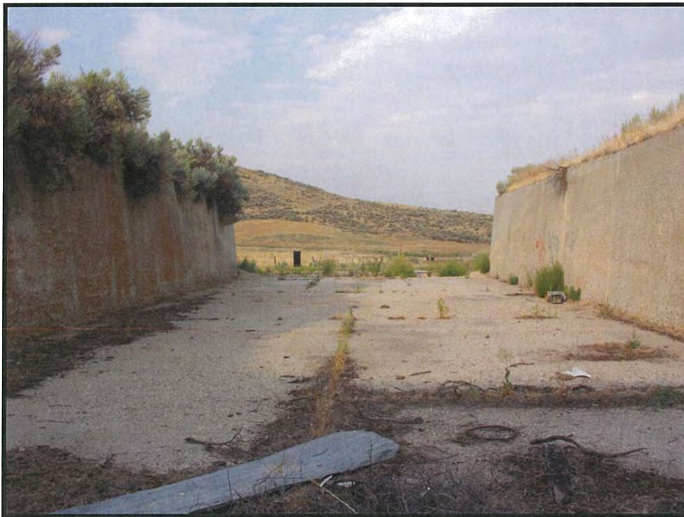
Figure 52. Feature 12, Silage Pit, viewed to the southwest (DSCN4184; 06/18/2016).
