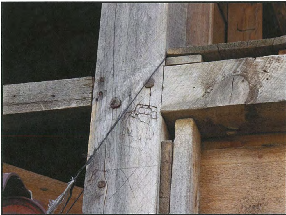
Figure 18. Feature 2, Horse Barn, mortise and tenon peg construction detail (DSCN4210; 06/18/2016).
