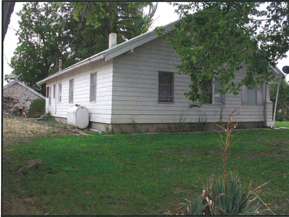
Figure 27. Feature 4, Dwelling, to the east, southeast (DSCN4224; 06/18/2016). Feature 5 in background.
