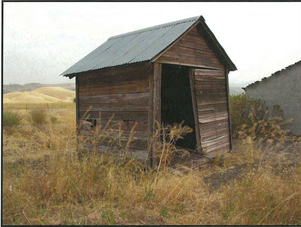
Figure 45. Feature 10, Brooder House, to the northeast (DSCN4269; 06/18/2016).
