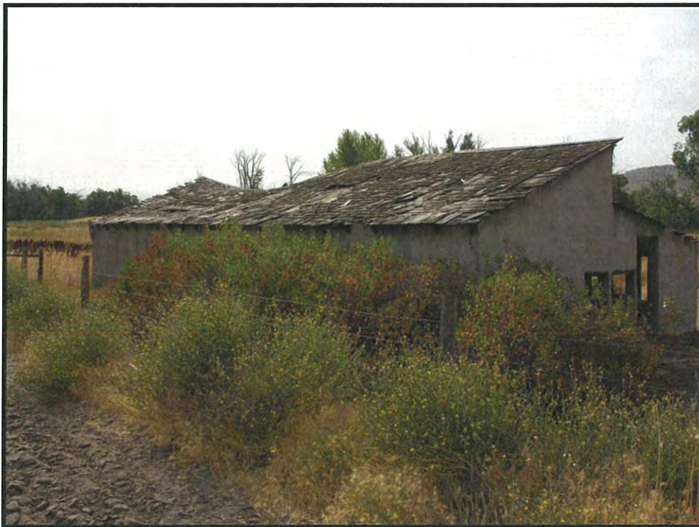
Figure 44. Feature 9, Chicken House, to the southeast (DSCN4262; 06/18/2016).
