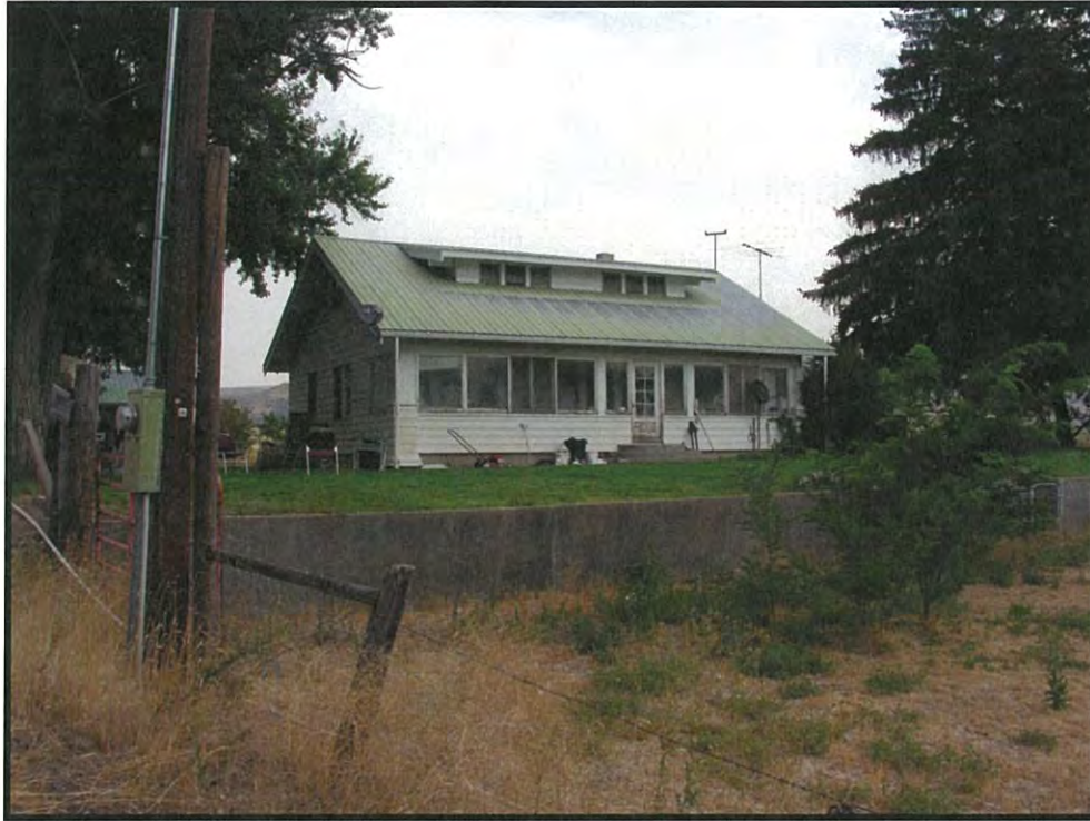
Figure 23. Feature 4, Dwelling, to the northeast (DSCN4228; 06/18/2016). Note four-foot retaining wall protecting the south side of the structure.
