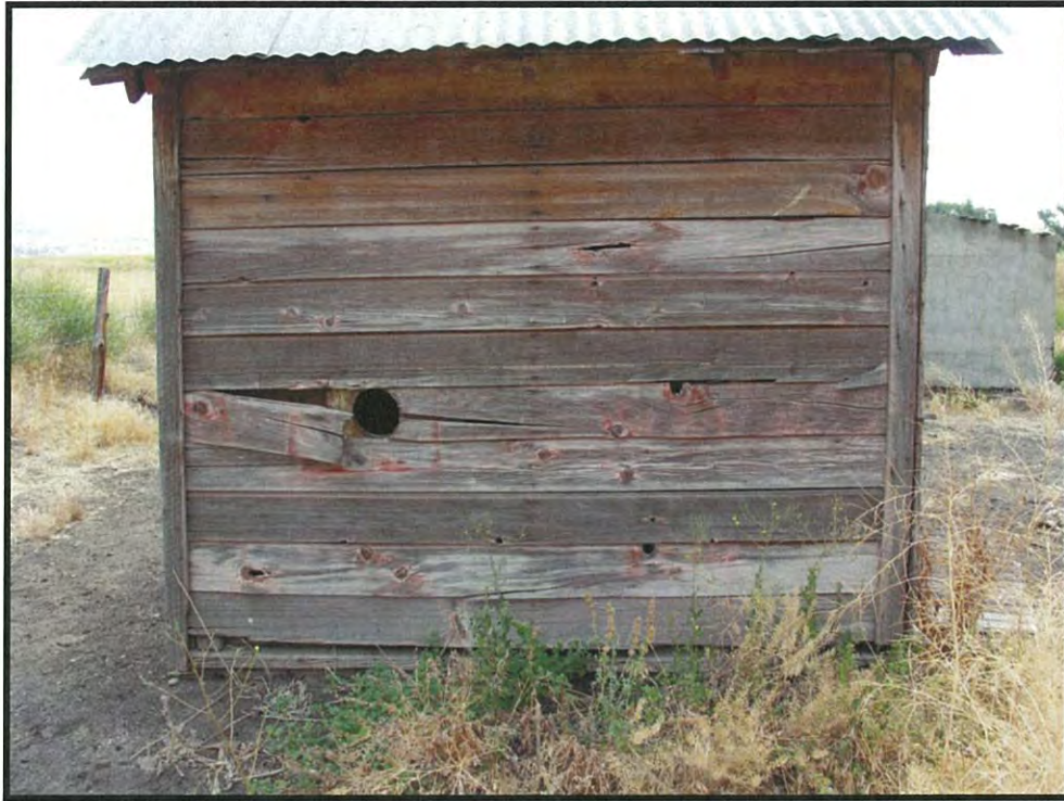
Figure 47. Feature 10, Brooder House, to east (DSCN4268; 06/18/2016). Note stovepipe hole for heater.
