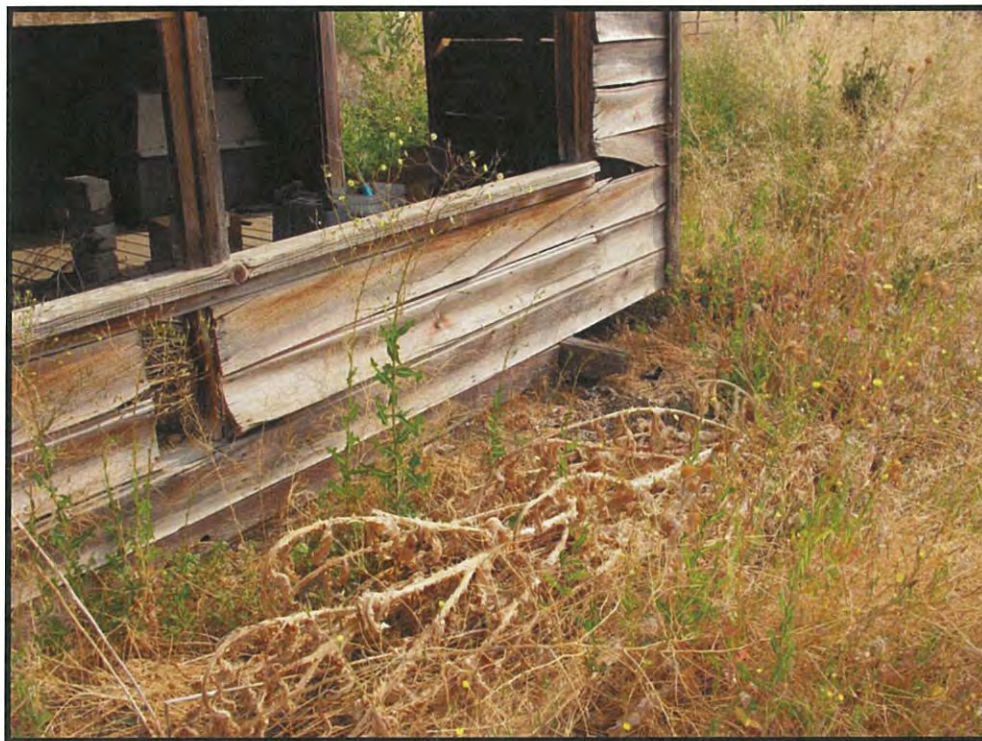
Figure 50. Feature 11, Relocated Chicken House, detail of chicken door and skid beam foundation (DSCN4281; 06/18/2016).
