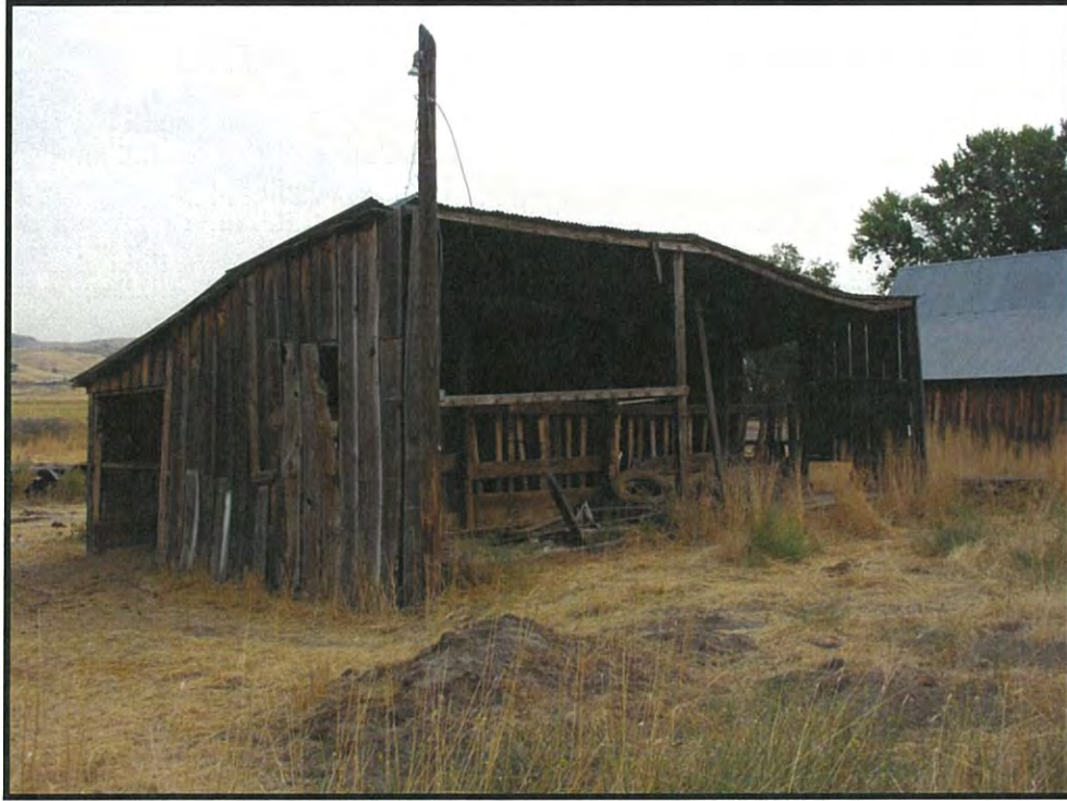
Figure 11. Feature 1, Dairy barn, to the northeast (DSCN4196; 06/18/2016).
