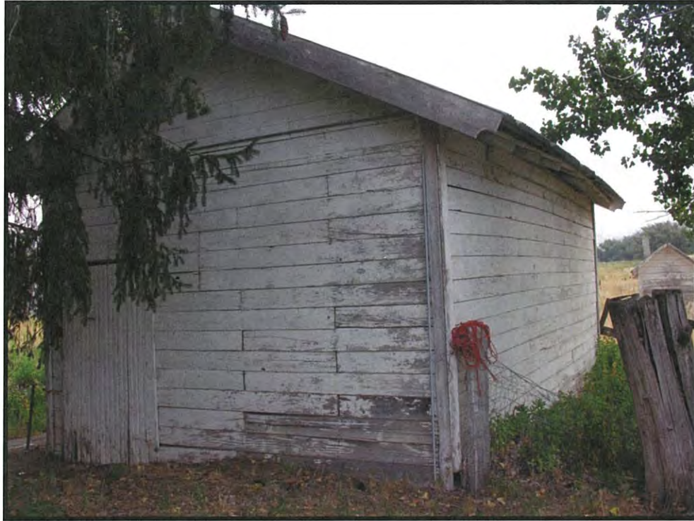
Figure 34. Feature 6, Machine Shop, to the northeast (DSCN4245; 06/18/2016).
