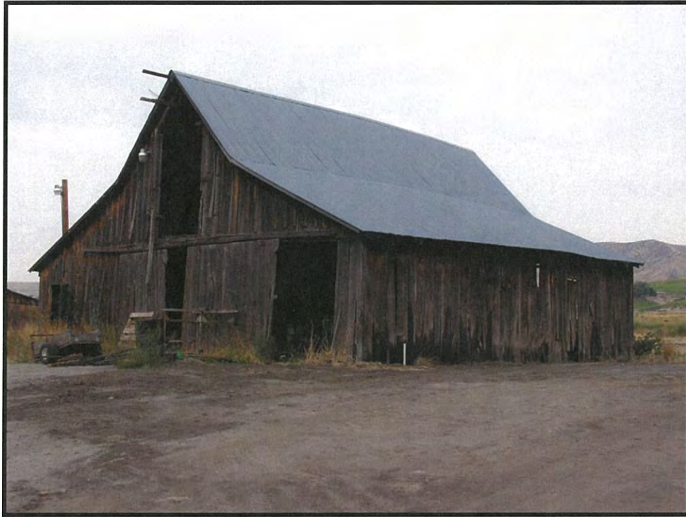
Figure 15. Feature 2, Horse Barn, to the northwest (DSCN4208; 06/18/2016).
