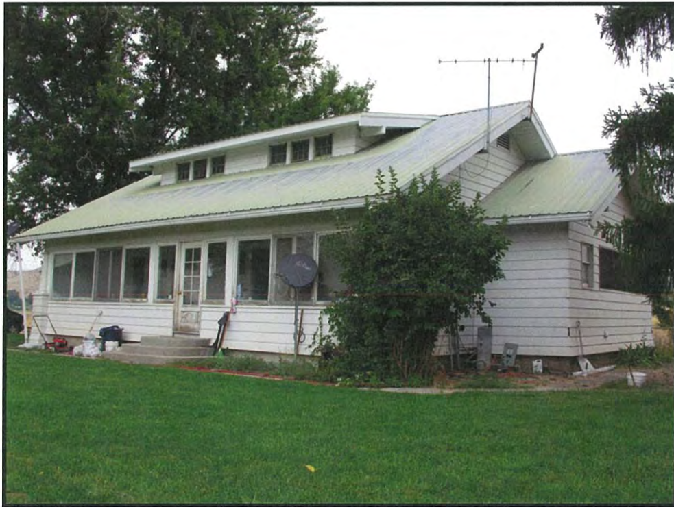
Figure 24. Feature 4, Dwelling, to the northwest (DSCN4231; 06/18/2016).
