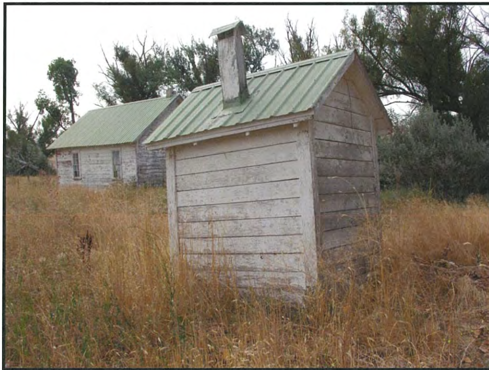
Figure 38. Feature 7, Privy, to the southeast (DSCN4250; 06/18/2016). Feature 8 in the background.
