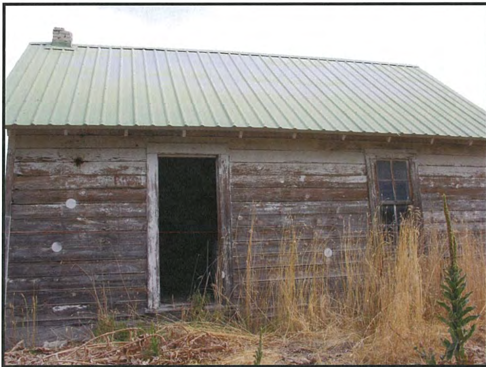
Figure 40. Feature 8, Bunk House entrance, to the north (DSCN4254; 06/18/2016).
