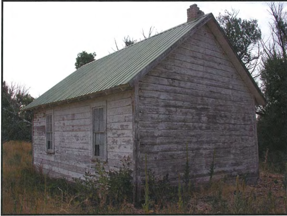
Figure 39. Feature 8, Bunk House, to the southeast (DSCN4251; 06/18/2016).
