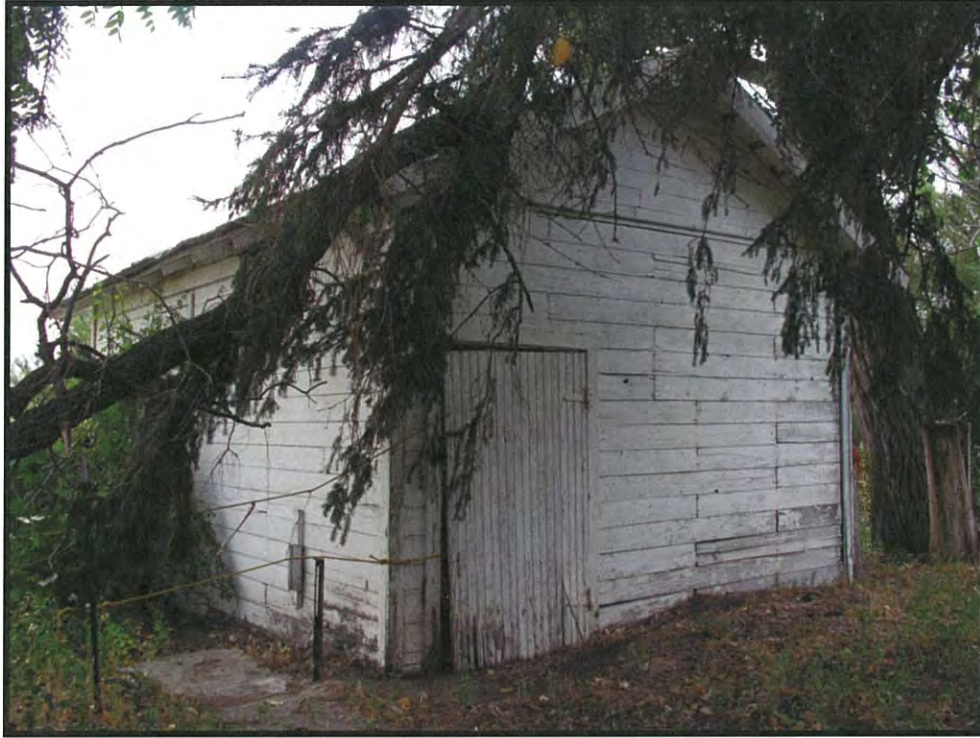
Figure 33. Feature 6, Machine Shop, to the southeast (DSCN4244; 06/18/2016).
