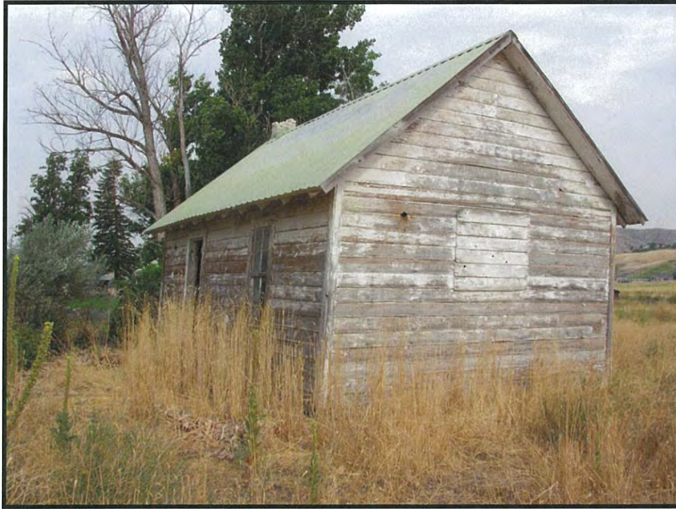
Figure 41. Feature 8, Bunk House, to the northwest (DSCN4255; 06/18/2016).
