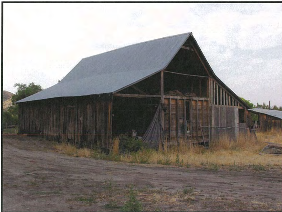
Figure 16. Feature 2, Horse Barn, to the southwest (DSCN4209; 06/18/2016).
