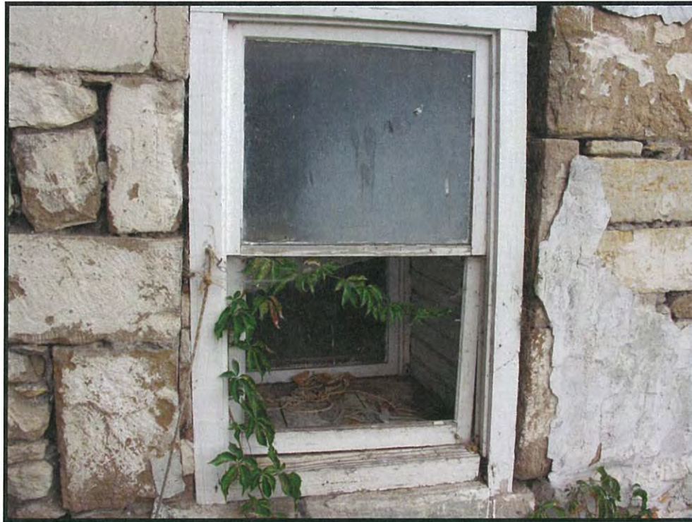
Figure 31. Feature 5, Cold House, window in east wall detail (DSCN4242; 06/18/2016).
